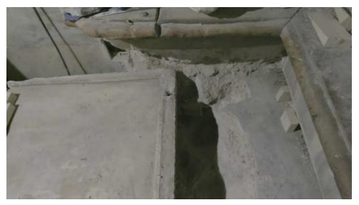
The top layer, upon which pilgrims have prayed for 450 years, was slid back, under which was another protective layer, of grey marble, which must be older still. This was badly damaged, revealing the bedrock of crumbly limestone underneath (above). After brushing away the dust of
